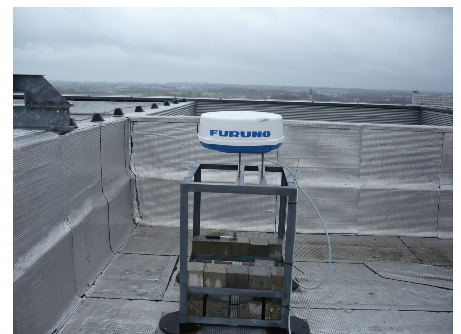
Rooftop view on the LAWR-CR (with the wall acting as clutter fence)
