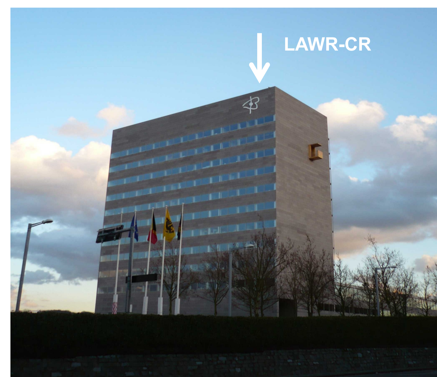
The Provinciehuis building (with LAWR-CR installed on the roof)
