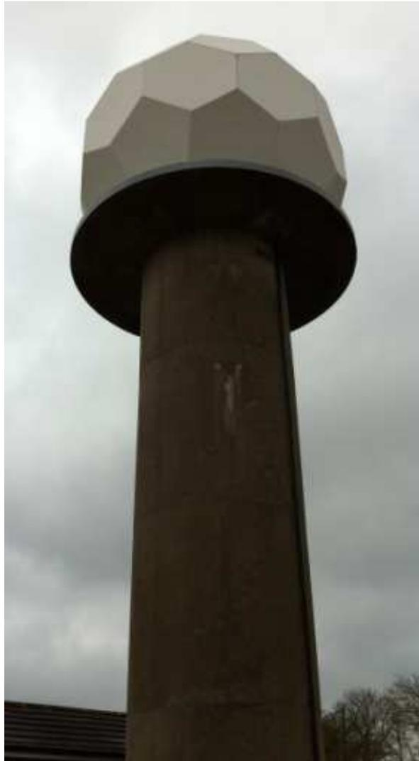
**Met. Office currently upgrading its C-band radar to dual pol.**
