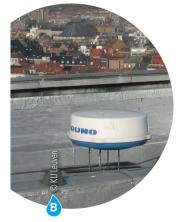
A Selex Meteor 60DX dual-polarisation X-band radar is being installed at the Cité Decartes campus in Champs-sur-Marne.
