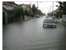
Figure 4: Street "Danton" in Livry-Gargan (23/08/2007) The water coming from this area is routed to the "Bassin de Poudrière"
