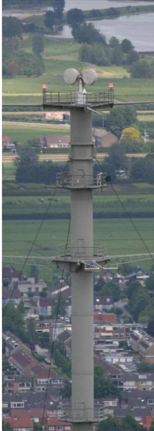
IDRA is mounted on top of the 213 m high meteorological tower.
